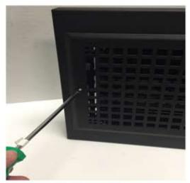
Place the Register Insert into the Baseboard Frame. You can install the damper control towards the top or bottom depending on the direction you would like the fins to point. Screw in the #6 x  $^{3}4$ " Black Head Screws into the Baseboard Frame using a #1 Phillips-Head Screwdriver.
