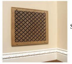
Step 6) Attach the grille cover with the included brass thumb screws
